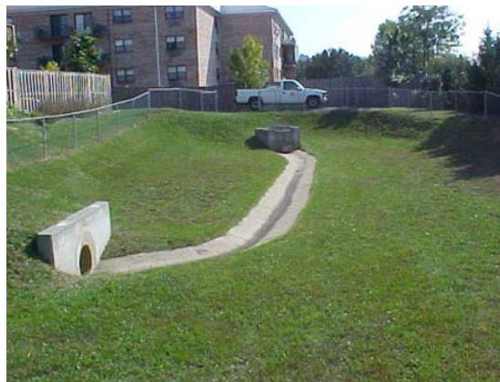
A traditional detention basin common in suburban New Jersey (Haberland et al.)
